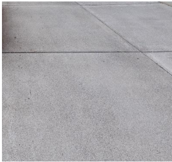
Plate 4-13 Example of concrete pavers/hardstanding
